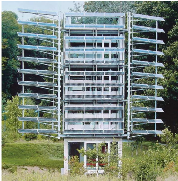
Fig. 5.5: Expo-Tower Wesertal Am Ohrberg: An example of BIPV with solar tracking [ 50 ]
