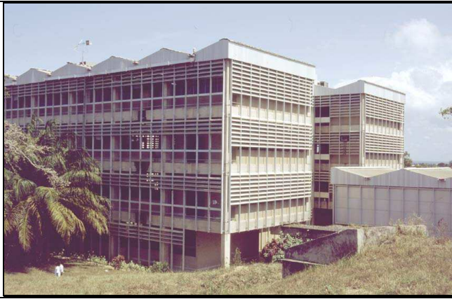
Fig. 5.23(a): The COET main building with its old roof (as it looked in 2004)
