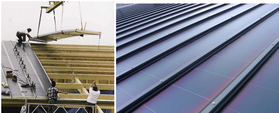
Fig. 5.7: Mechanised installation thin-film-on-metal BIPV roof and finished roof [51]
