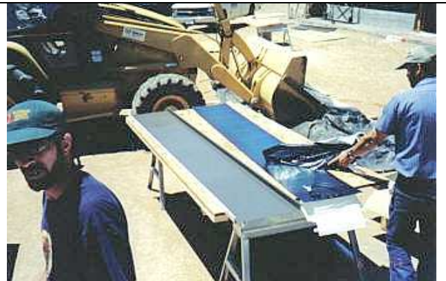
Fig. 5.19: Labour-intensive manual preparation of thin film PV sheet for roofing.
