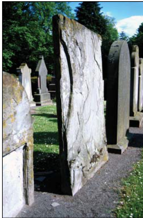
Figure 2.3: Delamination of a sandstone gravestone possibly resulting from frost action (from ICOMOS-ISCS, 2008).
