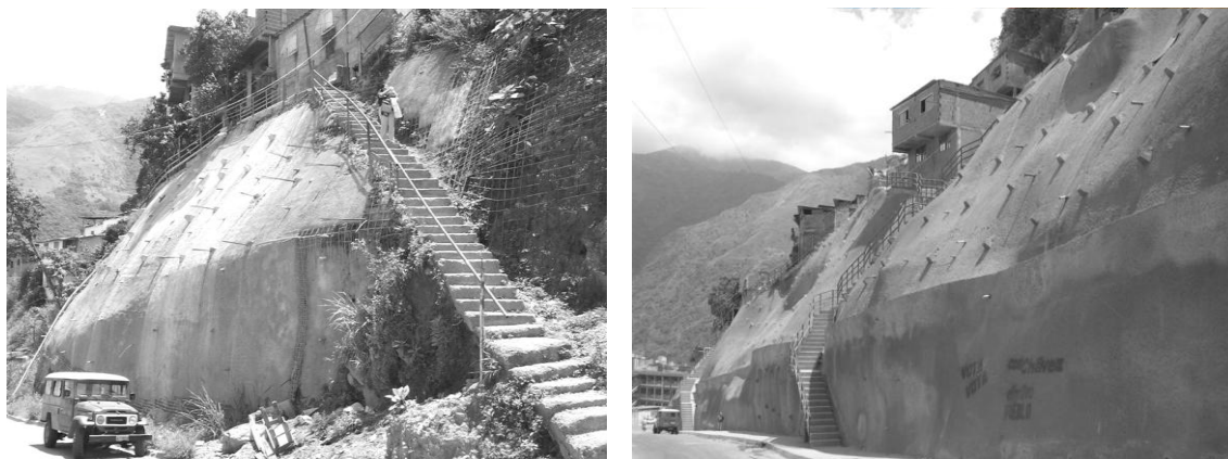
Figure 6.4: Retaining walls built by CAMEBA
