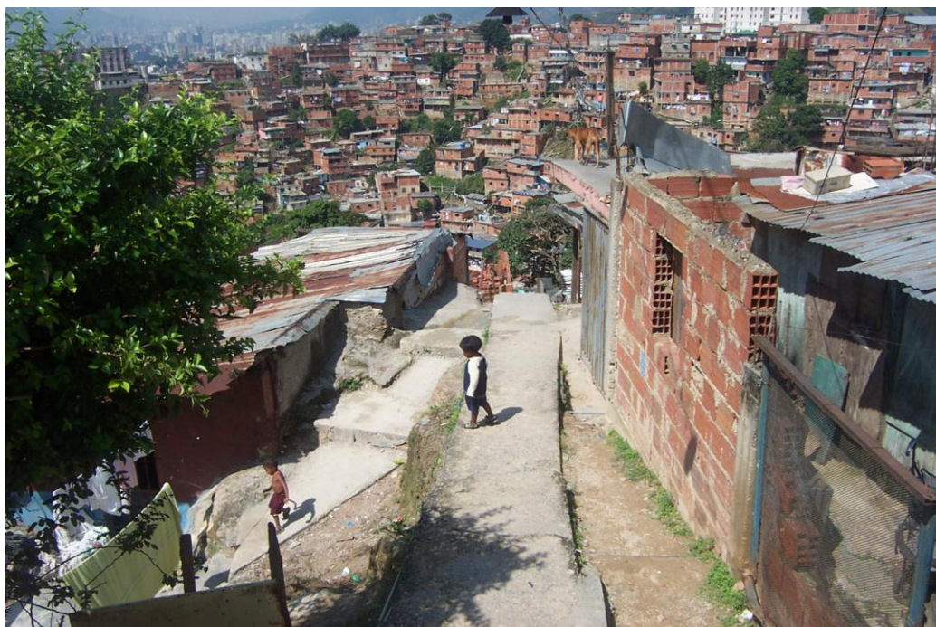
Figure 6.2: Dangerous state of the pedestrian movement paths
