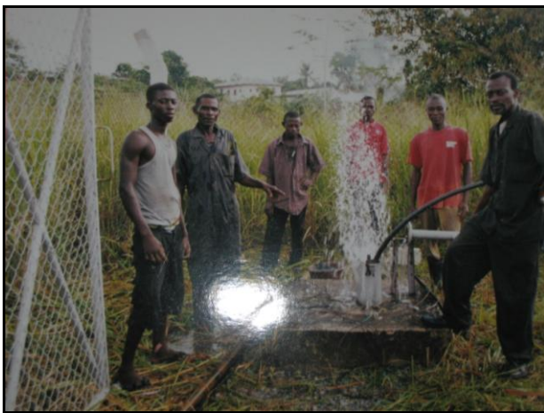
Picture 6.6 Staff of the JWS help in the process of re-developing one of the scheme’s boreholes as it is carried out by a contractor
