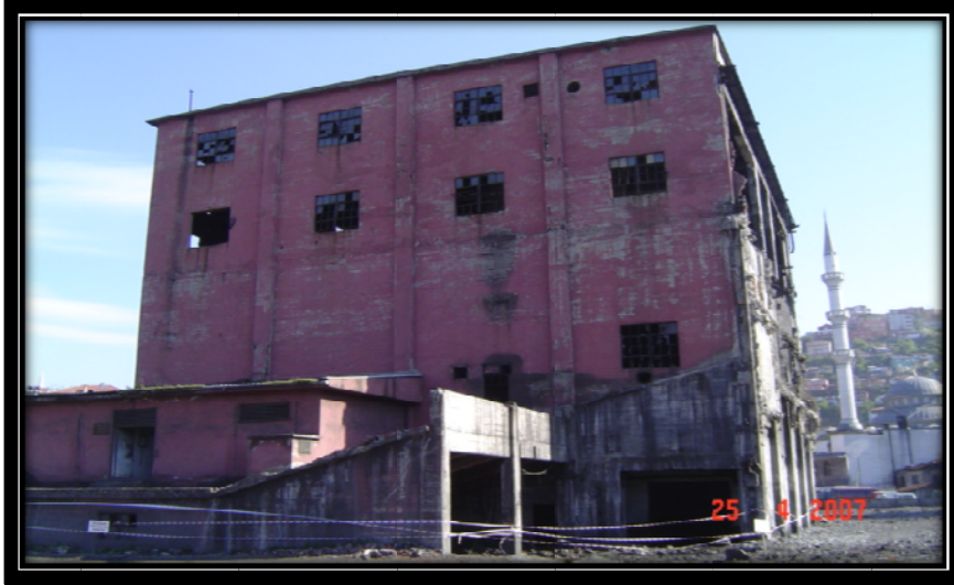
Figure-4.22: Old Coal Washing Area in Zonguldak
