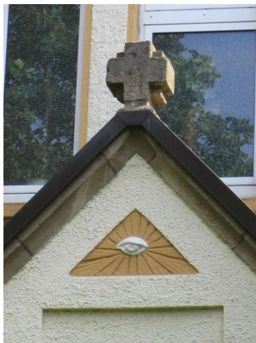
Abb. 5 – Giebfeld Portalvorbau (Detail) [2005]
