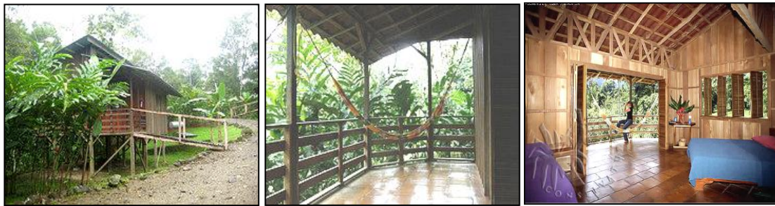
Figure (5.3): View of outside and inside the ecolodge cabins. Source: http://www.selvabananito.com/Cabins.html .
