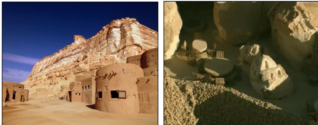
Figure (9.25): Exterior views of Adrere Amellal Ecolodge. Source: http://www.kiwicollection.com/hotel-detail/adrere-amellal-desert-lodge and image taken by the author.
