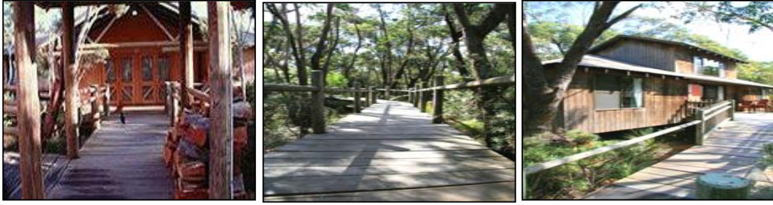
Figure (5.6): The wooden walkways placed above the ground. Source: http://www.jembyrinjahlodge.com.au
