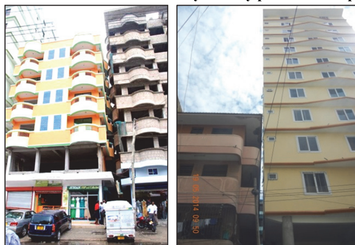
Figure 6.5: Encroachment towards boundary lines by private developers in Block 66
