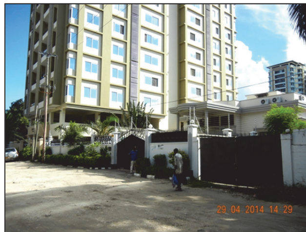
Figure 8.2: Building setbacks of new building vs an old one along Maweni Street
