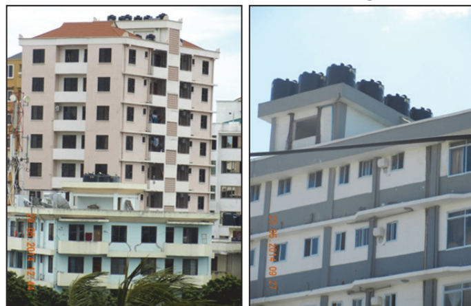
Figure 5.16: Raised water tanks as water shortage shock absorbers
