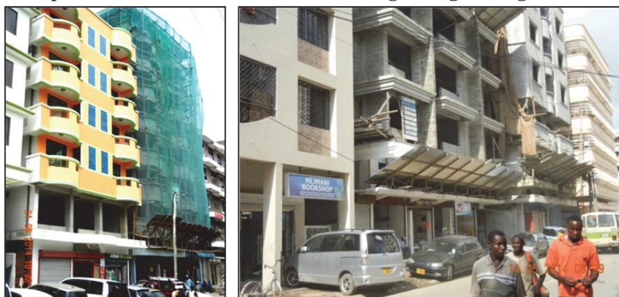
Figure 5.8: Shops in use in under-construction buildings along Mkunguni and Lindi Streets
