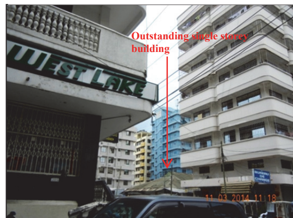
Figure 5.3: Demolition and redevelopment along Livingstone Street
