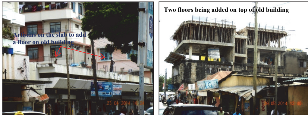
Figure 5.4: Vertical extension along Sikukuu and Kirk Streets
