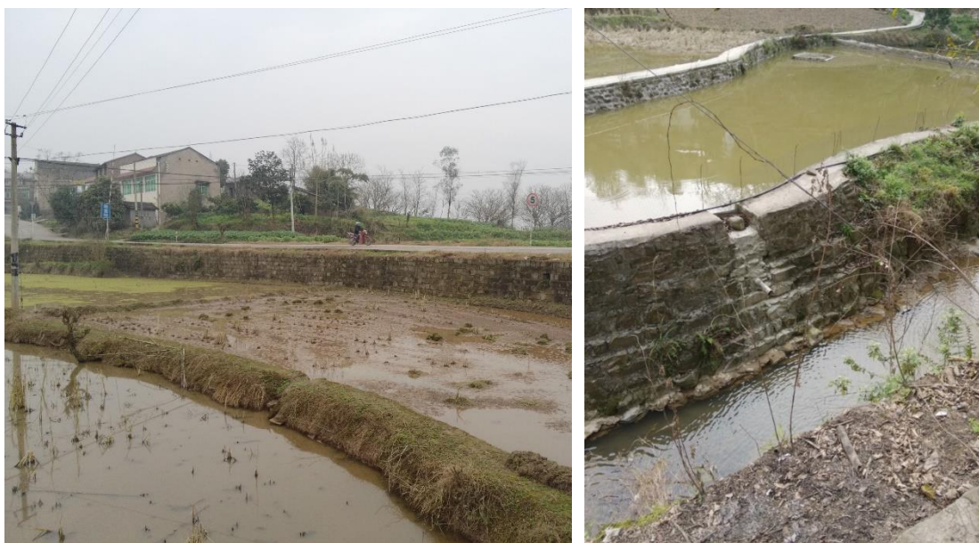
Figure 6.8 (left) & Figure 6.9(right) Modernized water control infrastructures.
