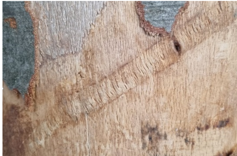
Fig. 3: Local fiber buckling in the bending compression zone
